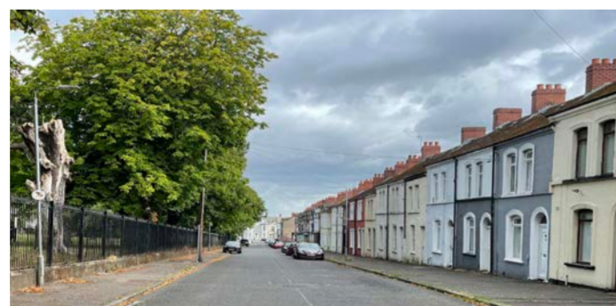
A derelict house opposite Woodvale park
